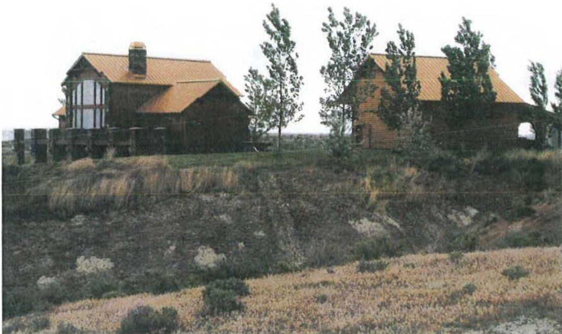
The east 500kV line is 250 feet west of this home.
