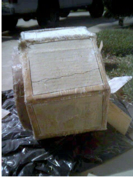
FIGURE 6. VIEW OF CRACKED CONCRETE UPPER SIDE PIPE WALL
